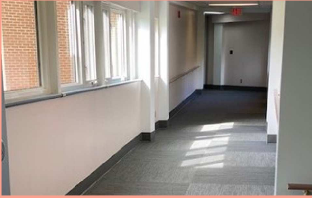
First Floor Carpet Replacement
