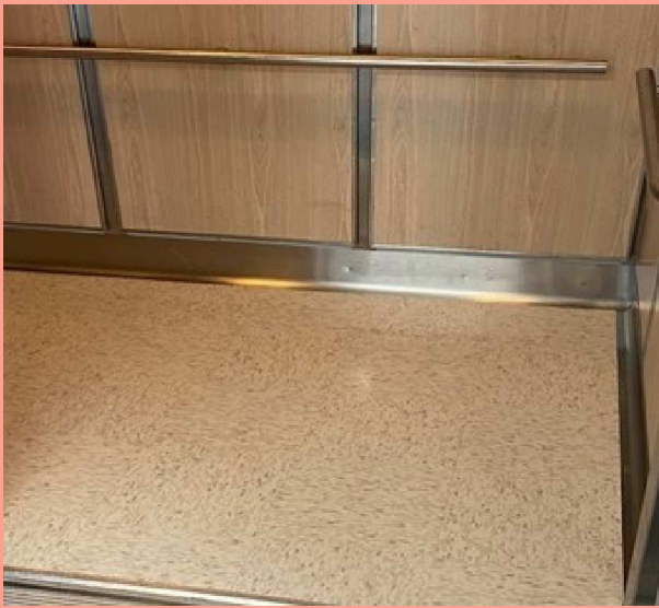
New Tile Flooring in Elevators
