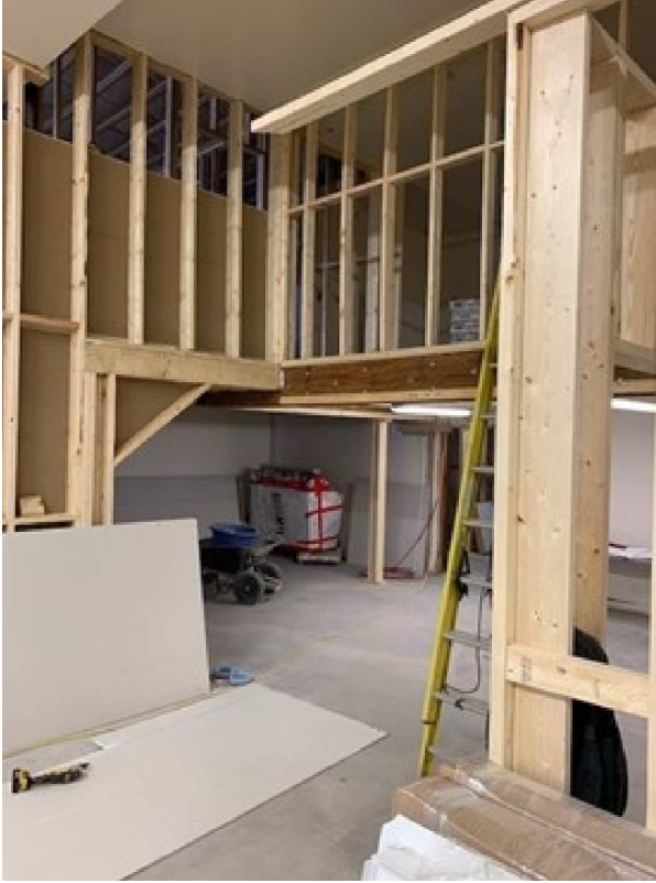
Looking from entrance common area into kitchen in back corner
